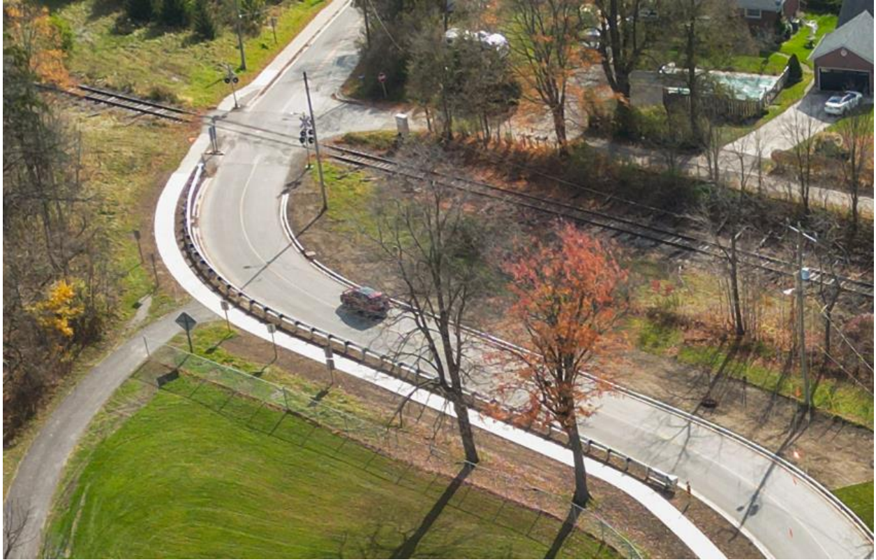
Figure 1 - Steel beam guide rail installed October 2024 between curb and sidewalk
